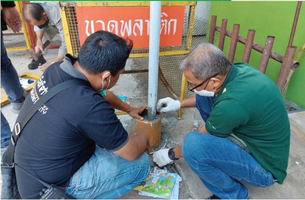
Improvement of Waste Sorting Plant
